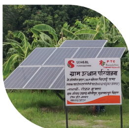
Land Mounted Solar Irrigation system, Muzaffarpur, Bihar
