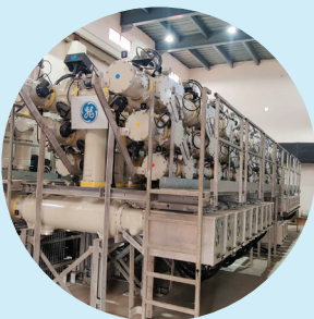
GIS installation and 220kV transmission connectivity at HPCL Visakhapatnam, Andhra Pradesh
